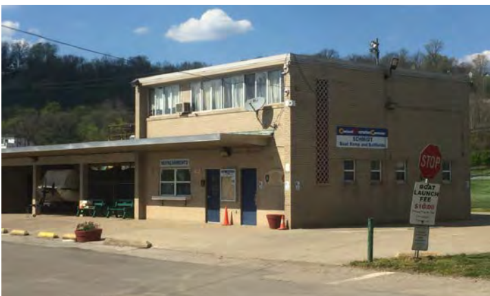
Top: The existing Schmidt Boat Ramp and Ballfields building could be expanded to include additional amenities such as kayak sales and rentals and camping amenities.
