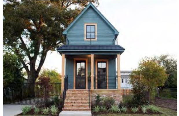
Example of a home built to bring the livable space out of the flood plain. Source: Pinterest.com
